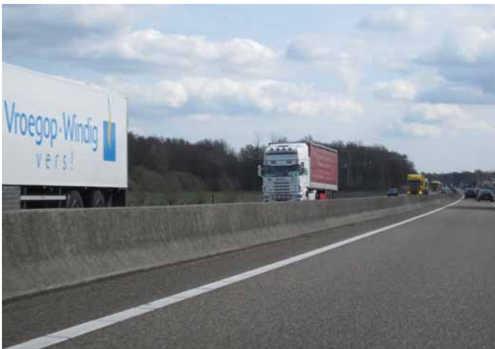
New Jersey barrier in the central reserve of a motorway
