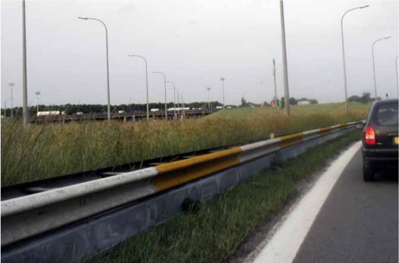
Example of a motorcyclist protection device, installed to an existing steel guardrail
