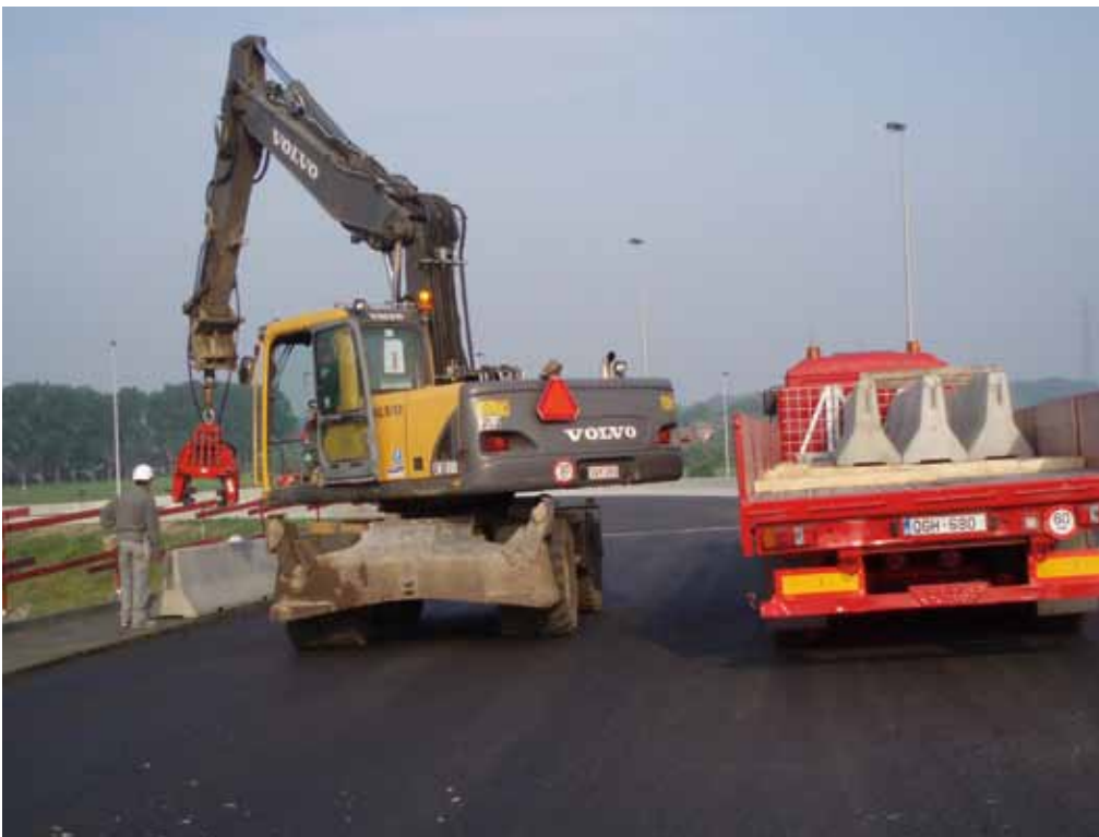
Installation of precast concrete barriers
