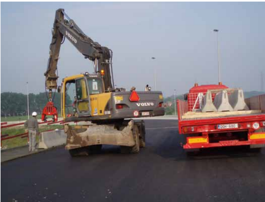
Installation of precast concrete barriers
