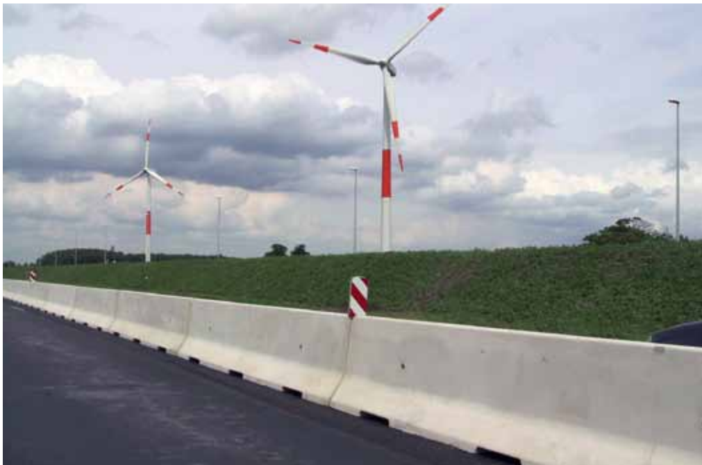
Precast barriers in a permanent and a temporary installation
