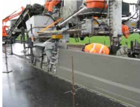
Surface mounted CSB installation
