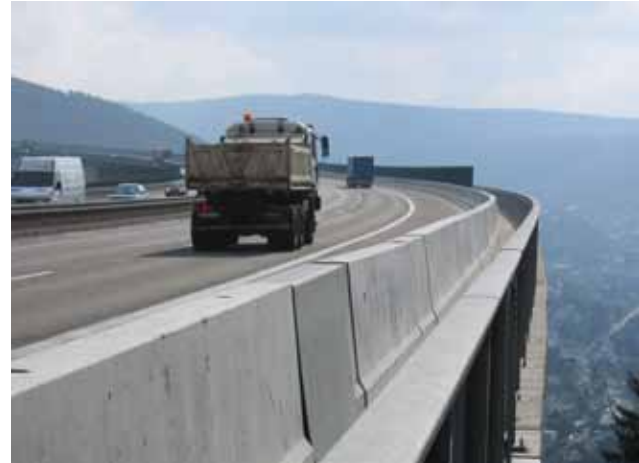
Example of a precast barrier with very high containment level (H4b) on a viaduct
