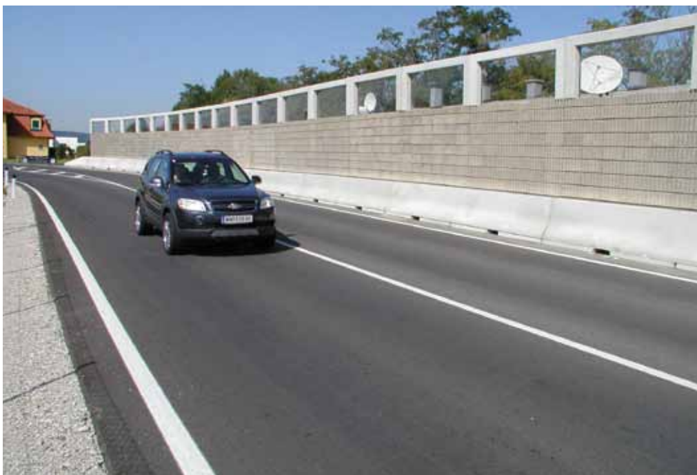
Example of a combined system of vehicle restraint system and noise barrier
